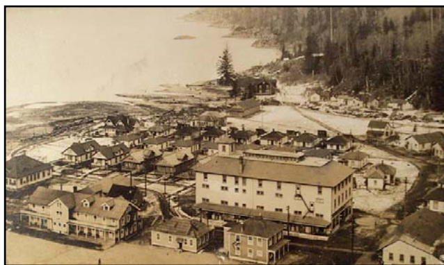
The Company Store was the largest non-industrial building in town.
